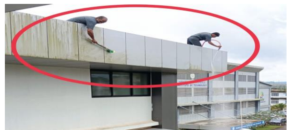
Figure 2. Manual Cleaning of Wall Panels in the college
